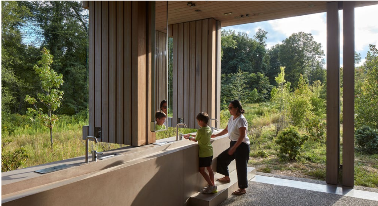
Storm King Restroom Pavilion (New Windsor, NY)
