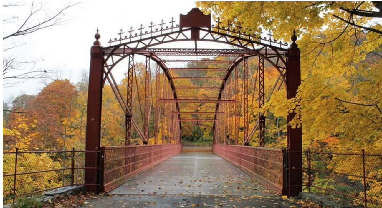
Lovers Leap Bridge (New Milford, CT)
